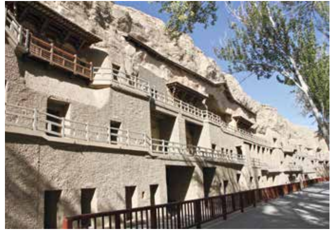
The Mogao Caves, cut into the mountainside
